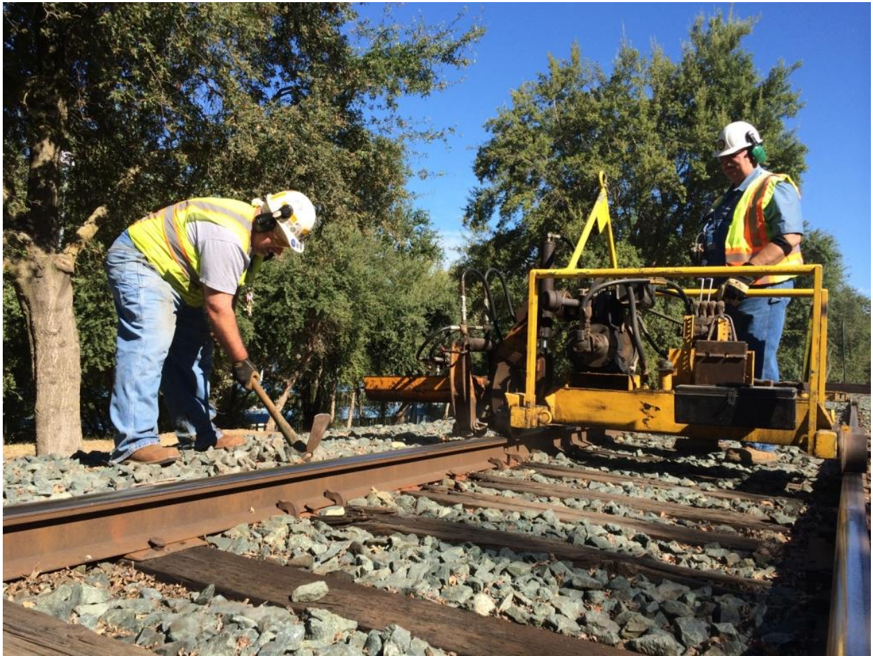
Dig, dig, dig. Mike F. and Chris try to keep the ties from disintegrating when being pulled
