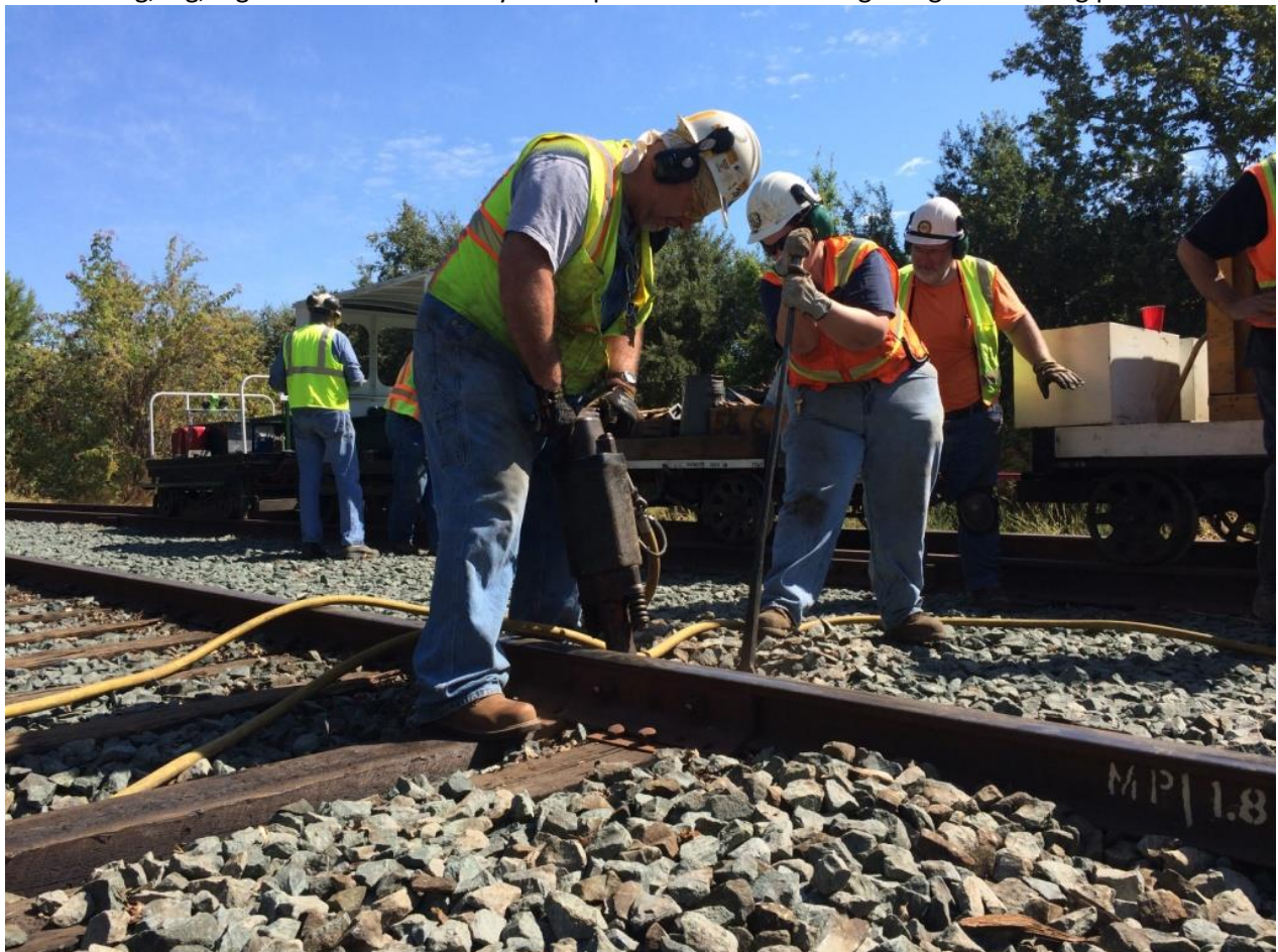
Mike F. with the pneumatic spiker while Heather nips the tie
