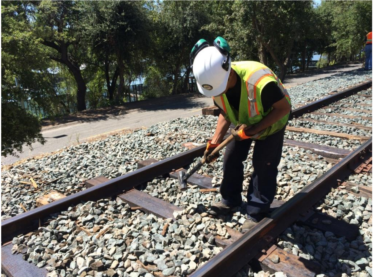
Josh pounds a rail anchor into place
