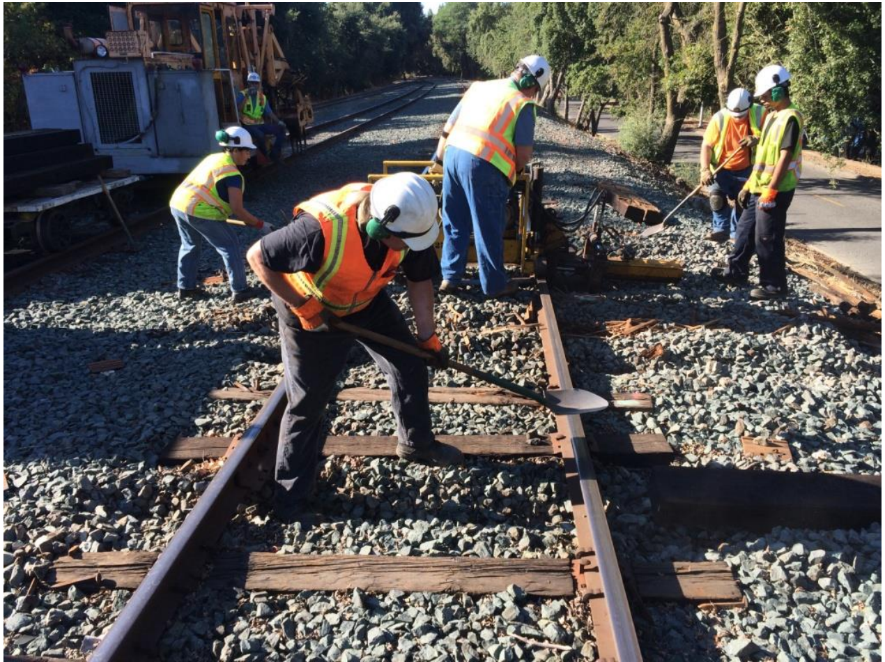
The MOW Team at work: Fred, Pam, Chris, Josh, and Frank prepping and pulling ties
