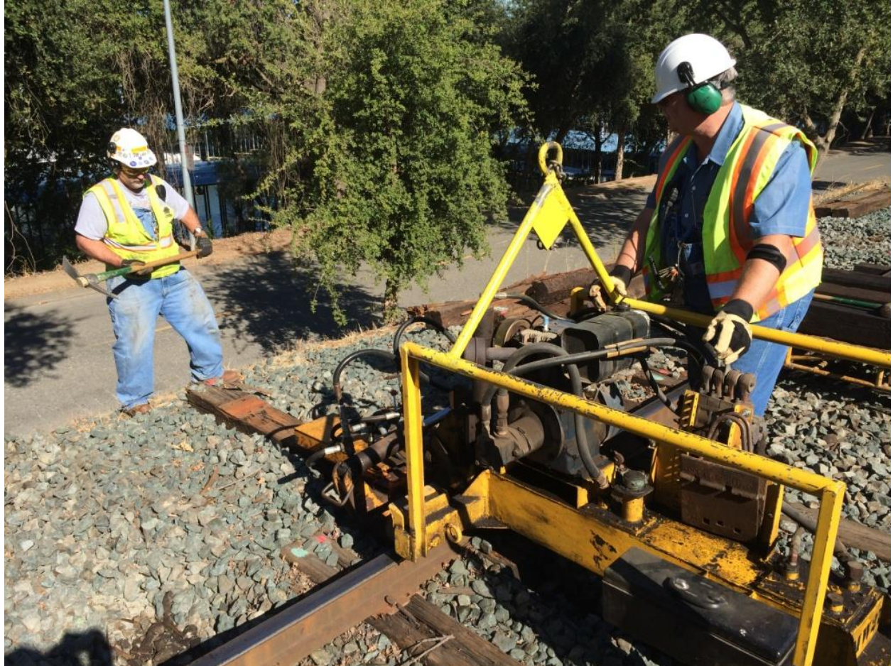
Mike F. and Chris work a rotten tie out from under the rails
