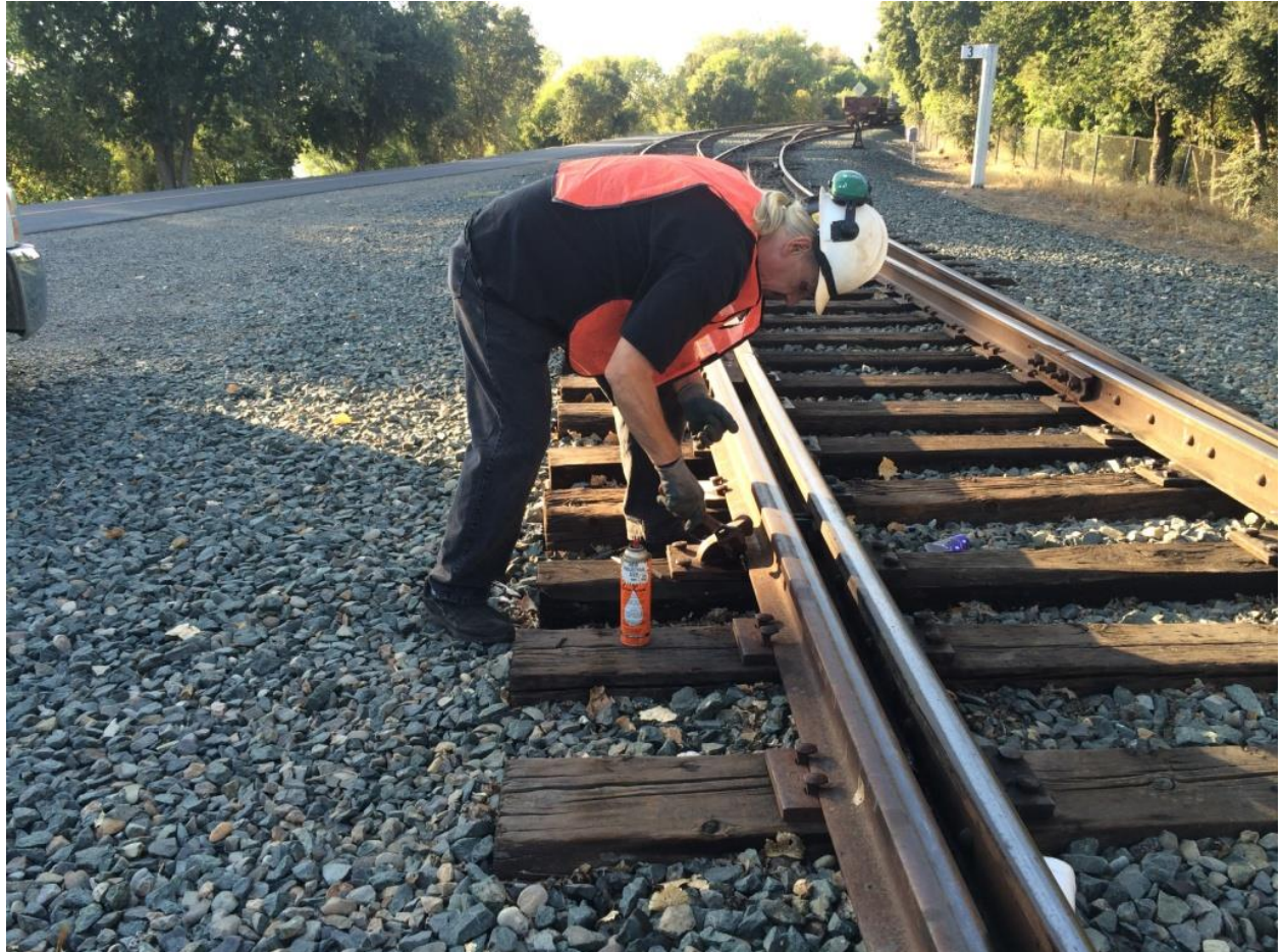
Fred loosening the bolts on the keepers in order replace the adjustable brace at Switch 20
